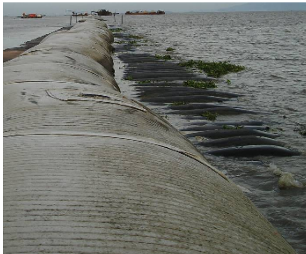
Figure 6: Geotextile tube used for coastal protection works
