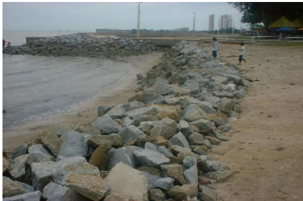
Figure 3: Rock revetment used for erosion
