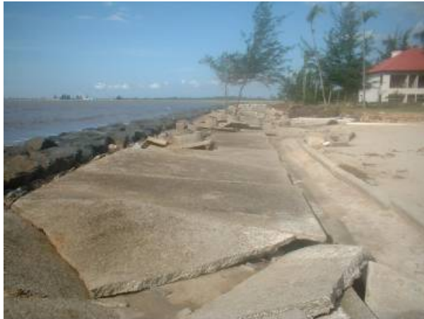
Figure 2: Concrete units used for erosion protection
