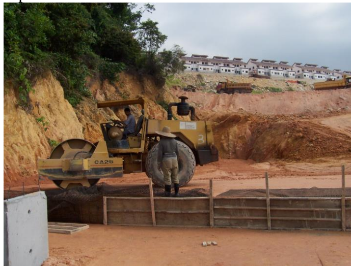
Figure 7: Compaction of backfill material in progress
