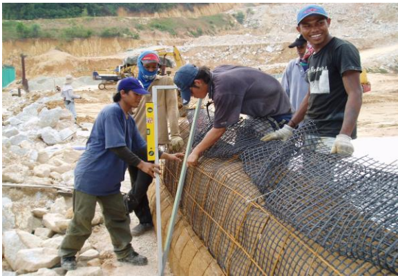
Figure 8: Installation of the wrap-around facing of the geogrid
