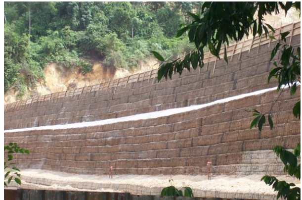
Figure 9: A completed section of the geogrid wall
