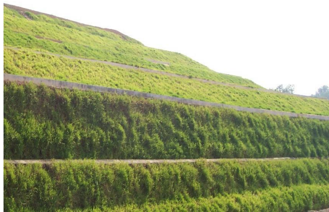
Figure 11: A view of fully vegetated facing
