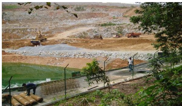
Figure 3: Rock-fill Base of Structure
